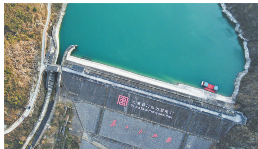
The Datang Bikou Hydropower Plant in Longnan city, northwest China's Gansu province. (PHOTO: XINHUA)
