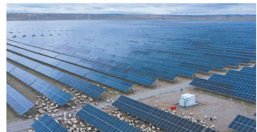
A flock of sheep roaming between solar panels at a solar photovoltaic power plant in Qinghai province. (PHOTO: XINHUA)
