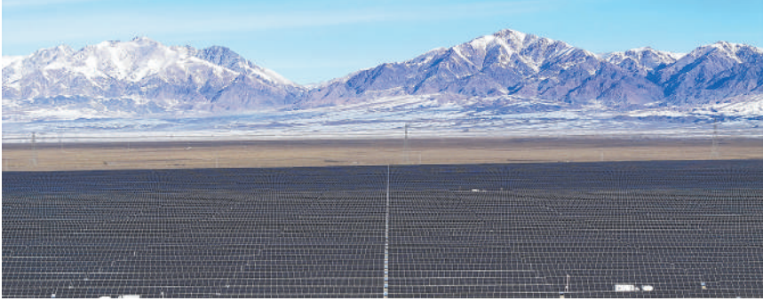
A corner of the Shichengzi photovoltaic industrial park in Hami city, Xinjiang Uygur autonomous region. (PHOTO: XINHUA)
