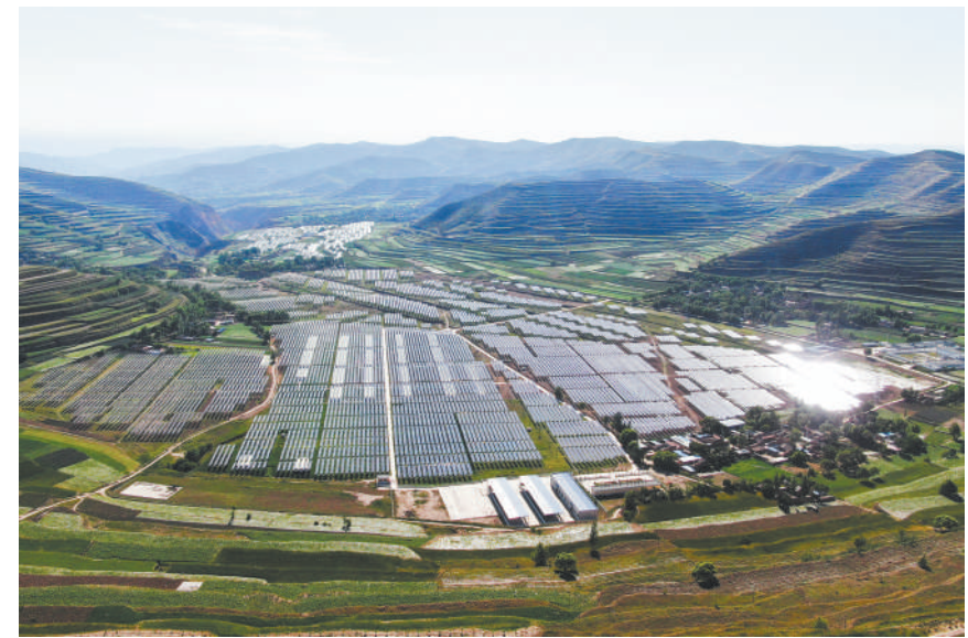
A centralized photovoltaic power station in Tongwei county, Gansu province. (PHOTO: XINHUA)
