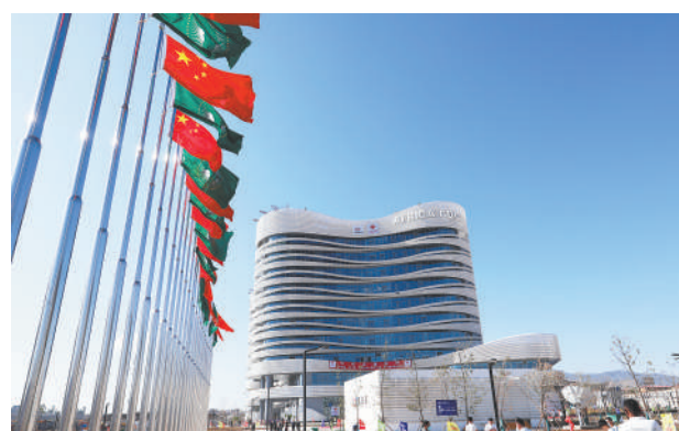
China-aided Africa Centers for Disease Control and Prevention (Africa CDC) headquarters project is completed in the southern suburb of Addis Ababa, capital of Ethiopia on January 11, 2023. (PHOTO: XINHUA)
