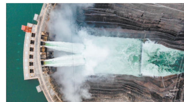
The Baihetan hydropower station, the world's second-largest in terms of total installed capacity, goes fully operational in the upper section of the Yangtze River in southwest China. (PHOTO: XINHUA)
