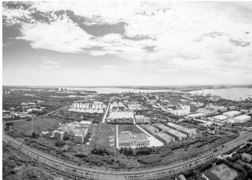
An aerial view of Hainan Yangpu Economic Development Zone, which is an important part of the Hainan Free Trade Port. (PHOTO: VCG)
