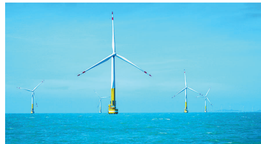
The Pinghai bay offshore wind power project in Putian, southeast China's Fujian Province. (PHOTO: XINHUA)
