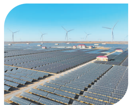
A solar power plant in Ningxia Hui Autonomous Region.
