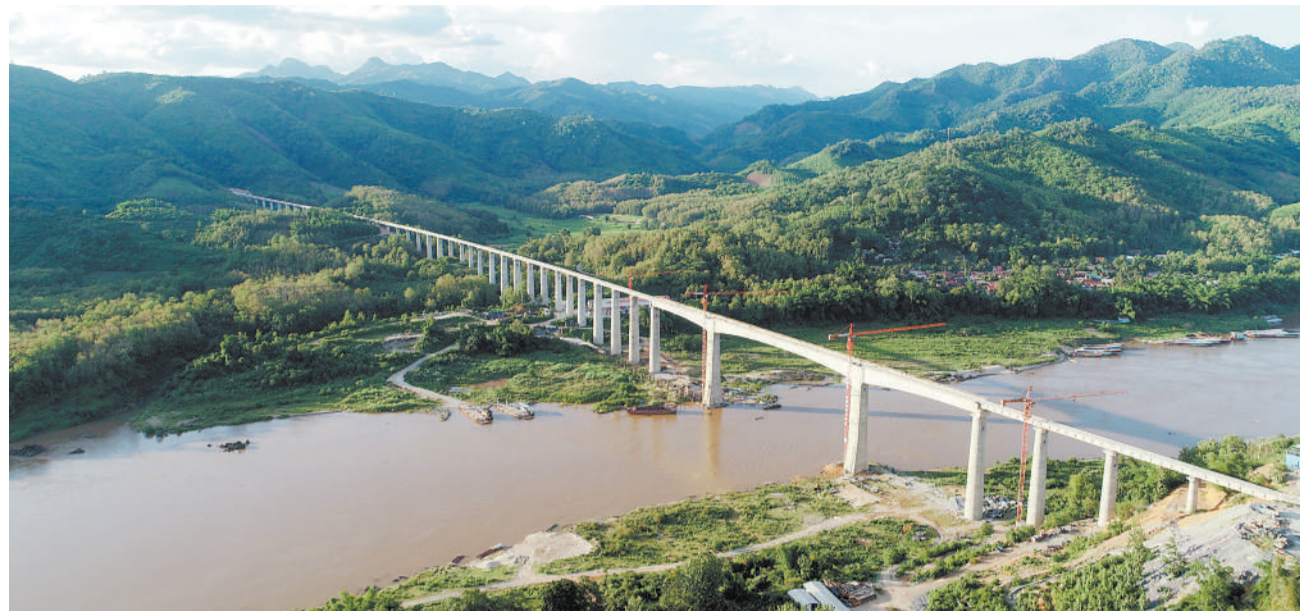
A view of the China-Laos Railway's Ban Ladhan Mekong River Super Major Bridge, located some 230 km north of Vientiane, Laos. (PHOTO: XINHUA)
